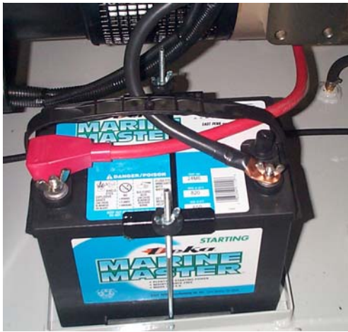
BATTERY CABLE INSTALLED
